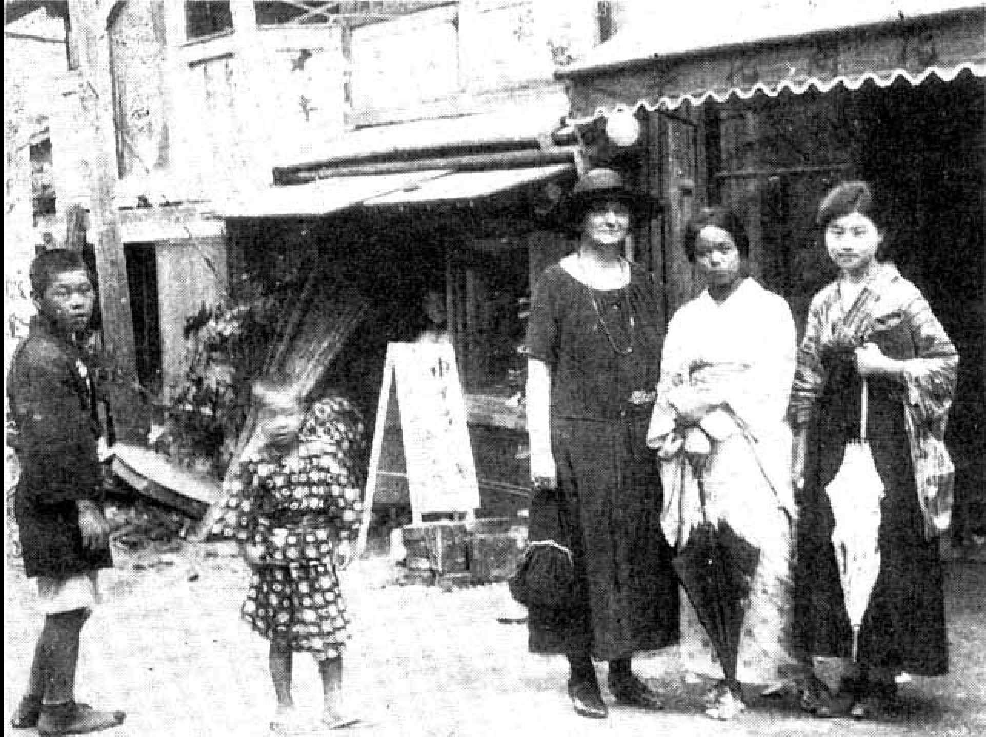
after the earthquake, Tokyo 1923
